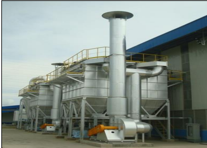
AIR PULSE TYPE BAG FILTER
